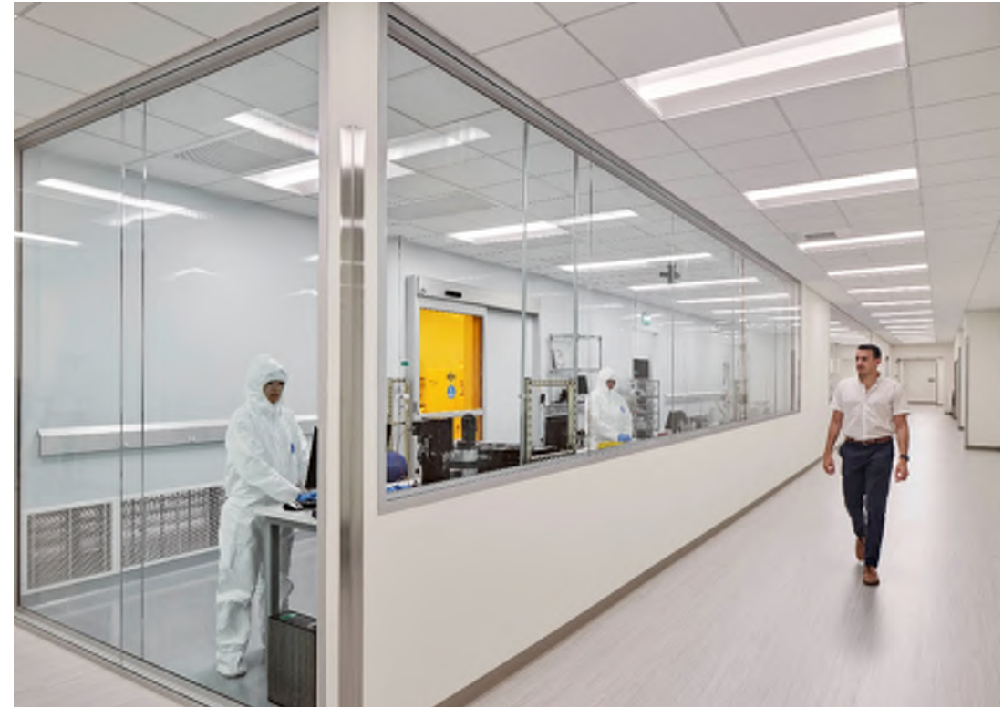
Public Corridor with View into Clean Room
