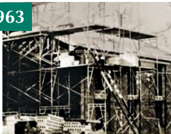
Construction of the Chestnut Hill campus begins
