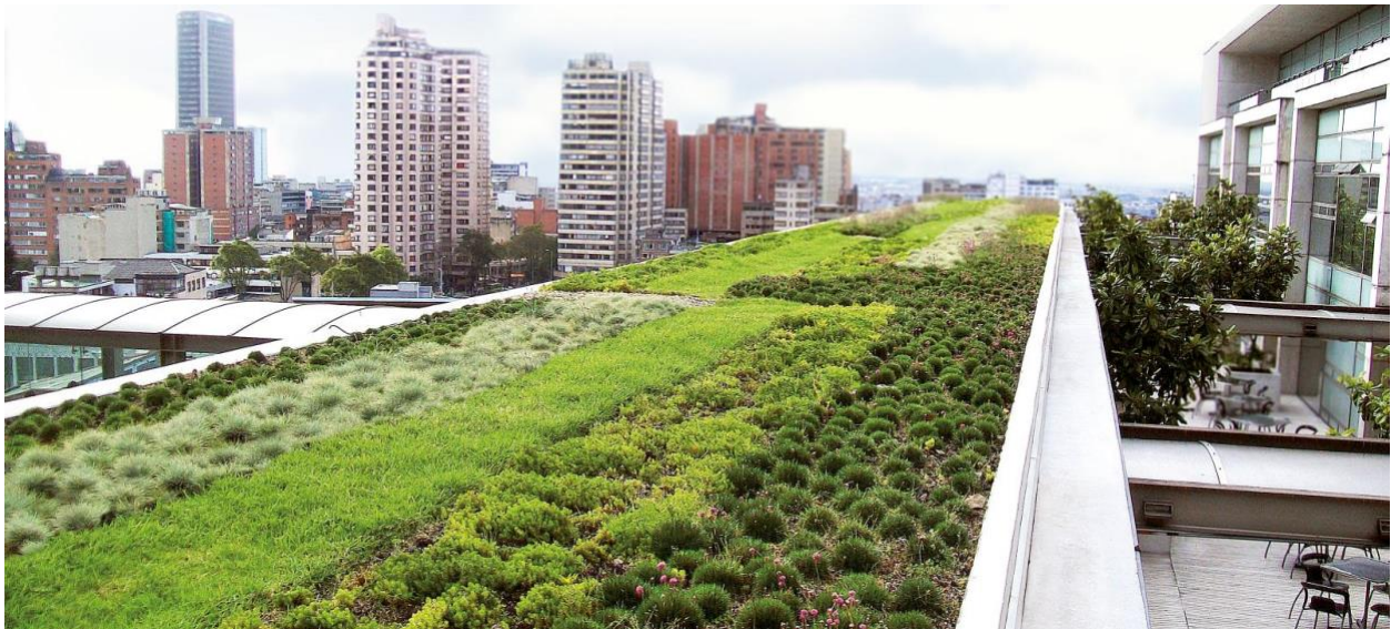
Figure 16: an example of an existing urban extensive green roof structure: This roof incorporates both sedum and grass species which is recommended for the new recreation center. (Stuckmann, Net Constructions)
